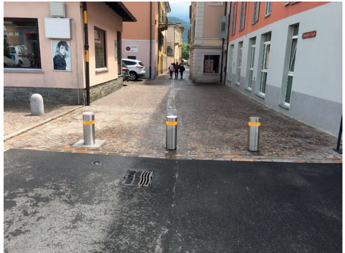
Retractable bollards 2 and fixed bollards Caslano
