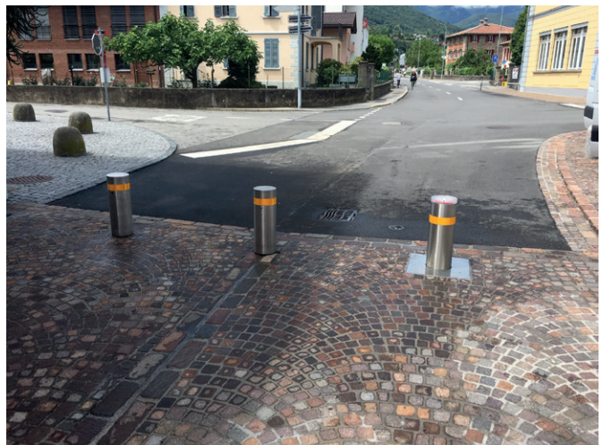
Retractable bollards 2 and fixed bollards Caslano
