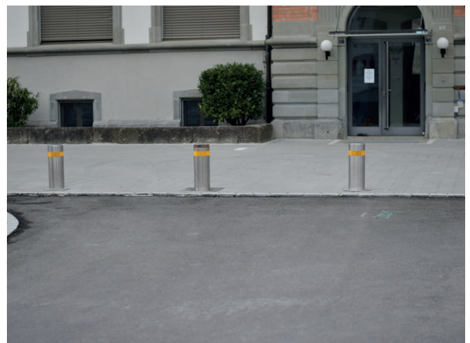
Fixed bollards and Retractable bollard school Thal
